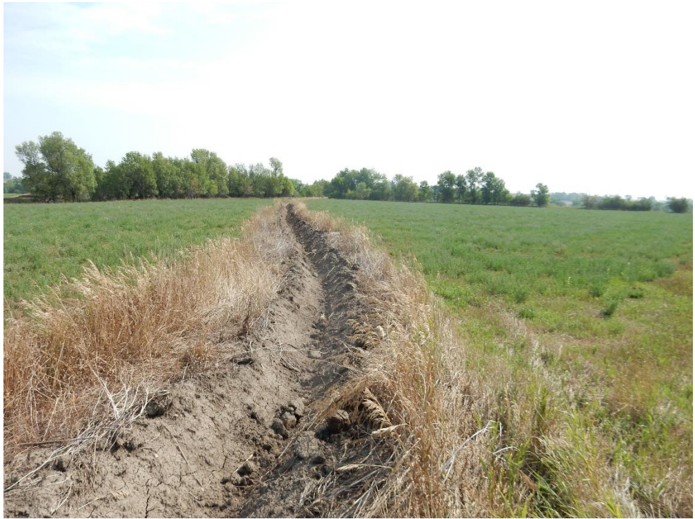
Figure 3-5. Typical On-Farm Earthen Irrigation Ditch Before Conversion to Underground Pipeline to Prevent Sediment Runoff.
