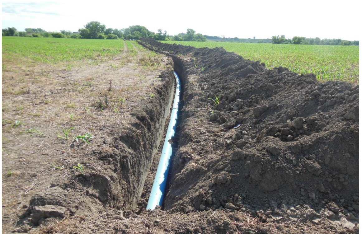
Figure 3-6. On-Farm Earthen Irrigation Ditch Conversion to Underground Pipeline to Prevent Sediment and Water Loss.
