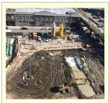
In-place treatment methods, such as soil solidification, may be effective for both contaminant immobilization and soil stabilization.
