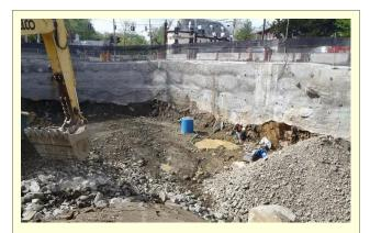
Early integration of remediation and redevelopment planning pays off. Structural support for contaminated soil excavation will become underground parking at a busy selected is based on situation-specific considerations, such as type of contamination, amount of contamination, depth to groundwater and extent of risk to human health or the environment. Additional cleanup might be necessary during the demolition phase to address issues, such as asbestos or lead-based paint.
