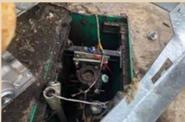
A properly functioning shear valve mechanism that closed completely after a tornado leveled a gas station and blew away the dispenser. Credit: EPA
