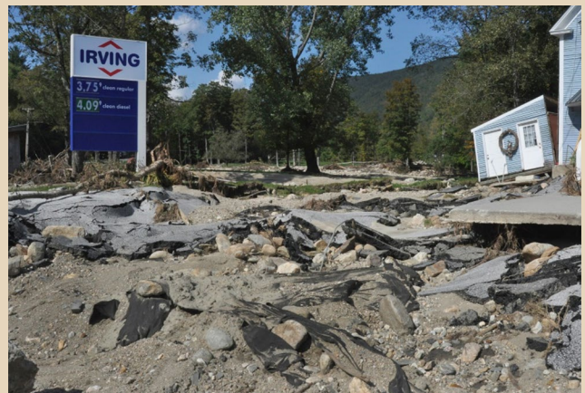
Blackie's General Store - Soil erosion and scour from Ottaquechee River flooding. Tropical Storm Irene - August 2011. Credit: New England Interstate Water Pollution Control Commission
