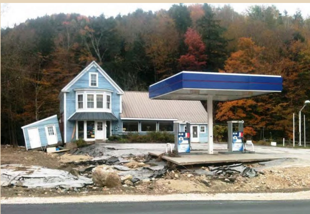
Blackie's General Store - Soil erosion and scour from Ottaquechee River flooding. Tropical Storm Irene - August 2011. Credit: New England Interstate Water Pollution Control Commission
