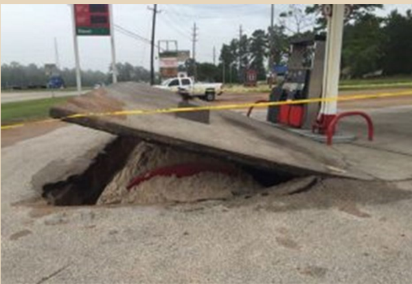
Examples of USTs affected by buoyancy. Hurricane Katrina, 2008. Credit: EPA
