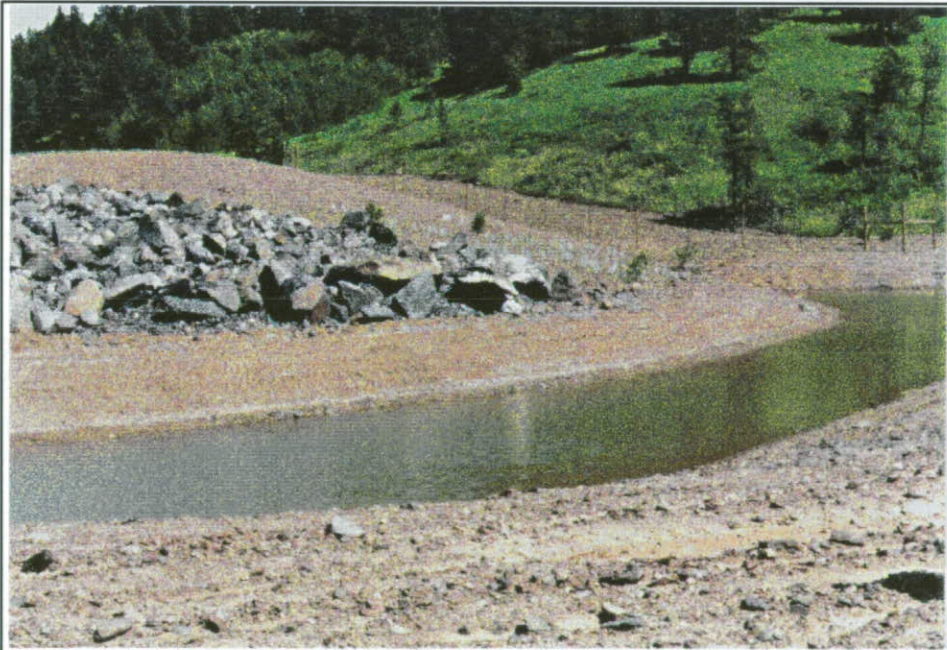
Photo 1.4 – Homestake created a pond and placed rock structures on the reclaimed Sawpit Waste Rock Depository for wildlife habitat.
