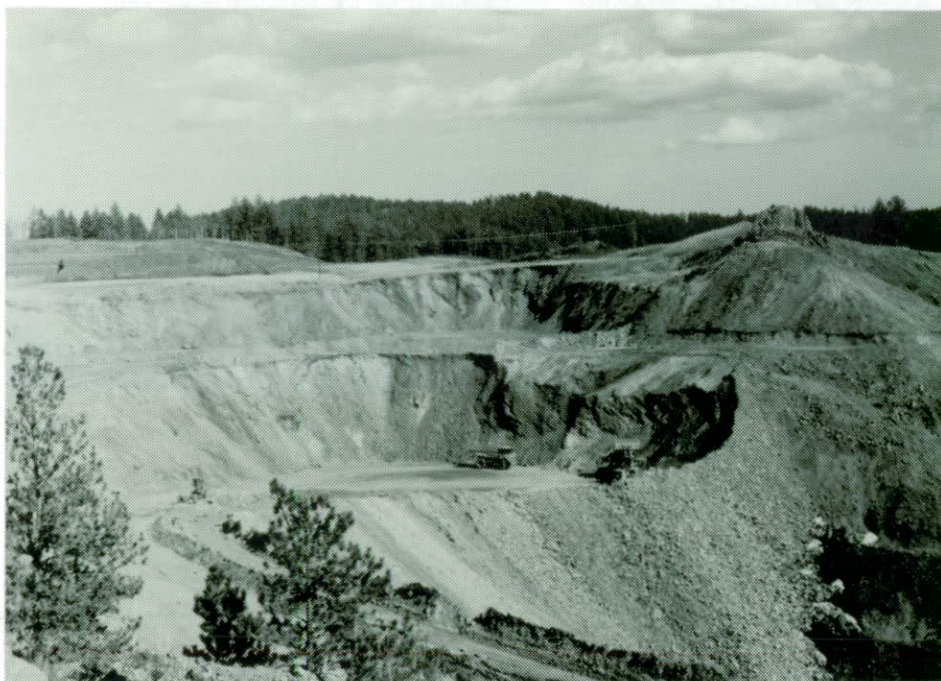
Photo 1.2 - Spruce Gulch Waste Dump as Waste Rock is Being Removed
