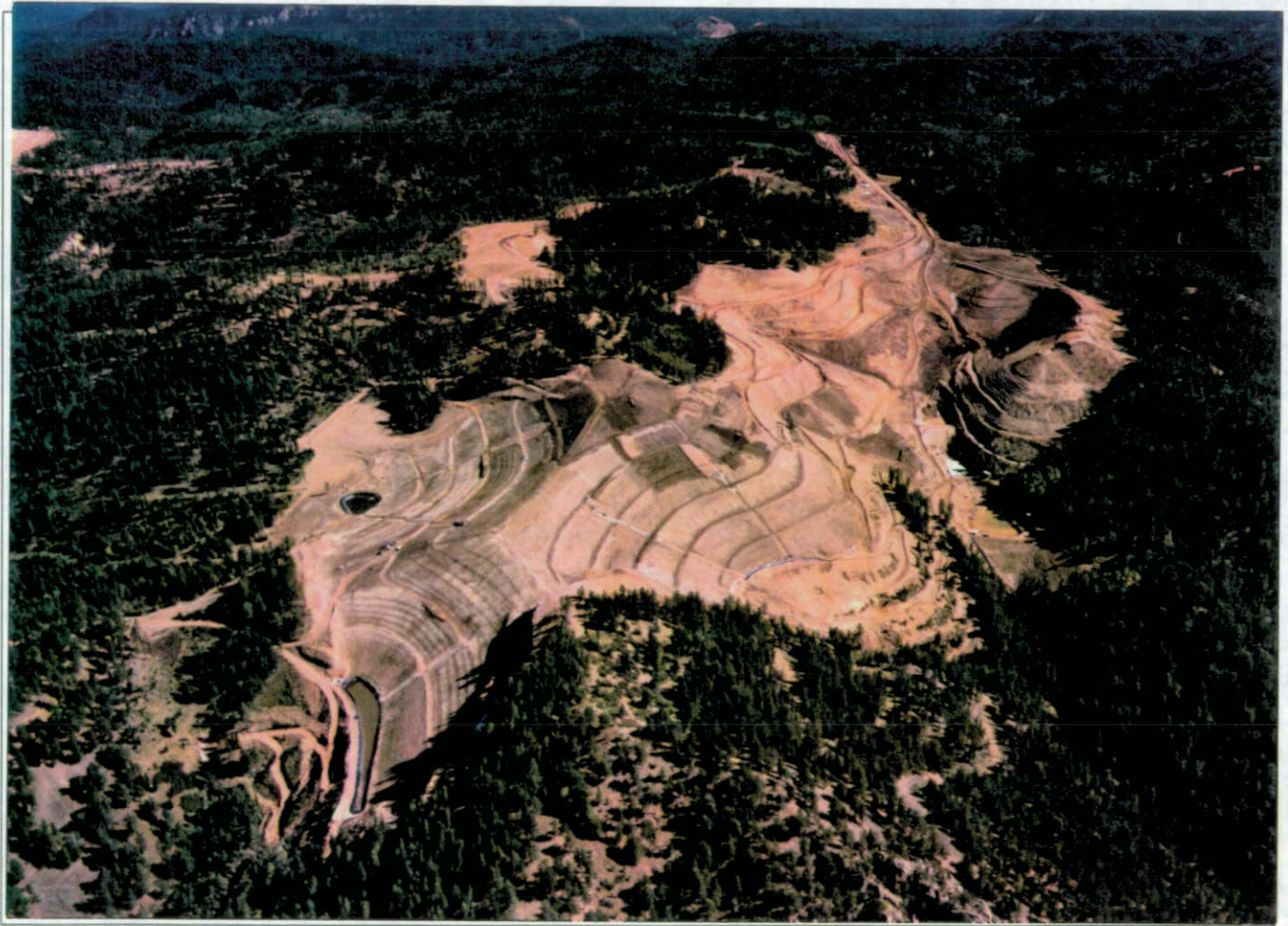
Photo 1.1 - Completed Richmond Hill Pit Impoundment (Photo courtesy of LAC Minerals)
