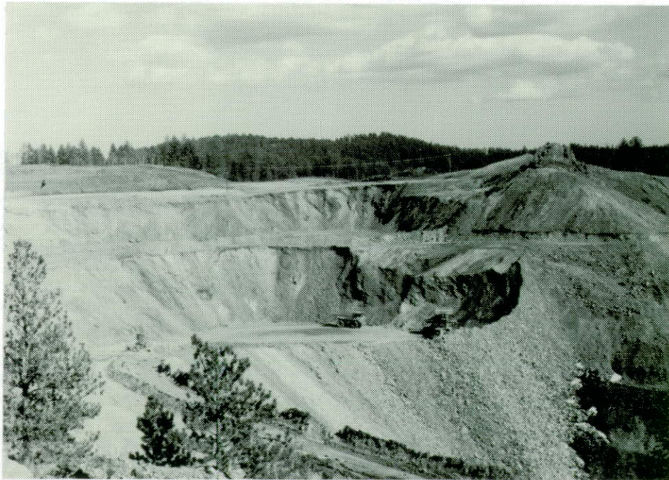
Photo 5 - LAC Contractors Removing Acid Generating Rock from Waste Rock Dump
